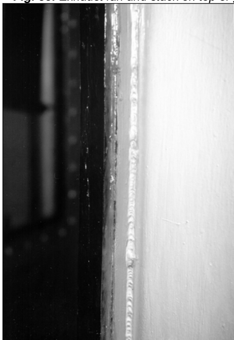
Fig. 90: Closeup of rubber seal around gas chamber door, also covered in vaseline when in use.
