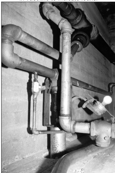
Fig. 94: Portion of plumbing and sewage system connecting chemical room to gas chamber.
